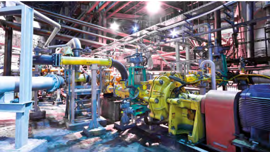
Slurry pumping station
